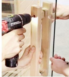
Door Handle Installation
