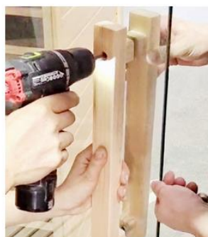
Door Handle Installation
