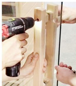
Door Handle Installation
