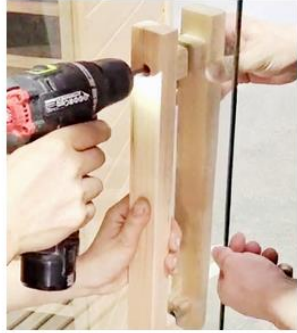
Door Handle Installation
