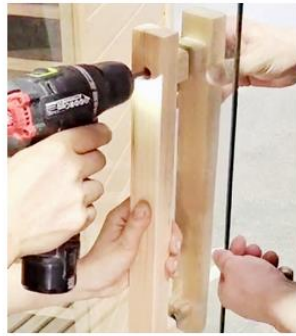
Door Handle Installation
